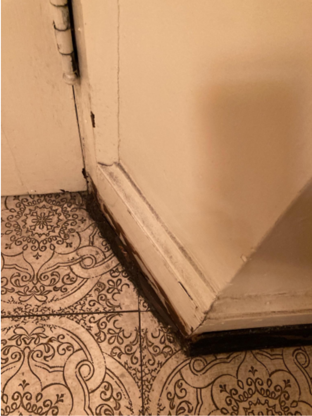
Floors and baseboards following cleaning on the 20th of July.
