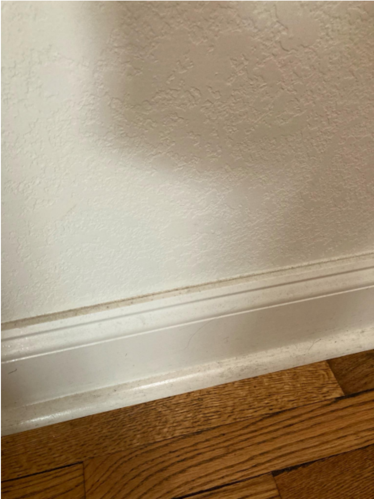
The baseboards after cleaning.
